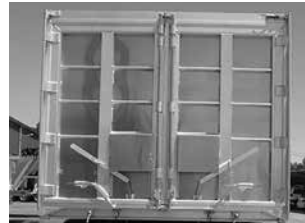
Door leaves with door lintel
